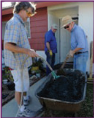
Mixing cement for the ramp.
